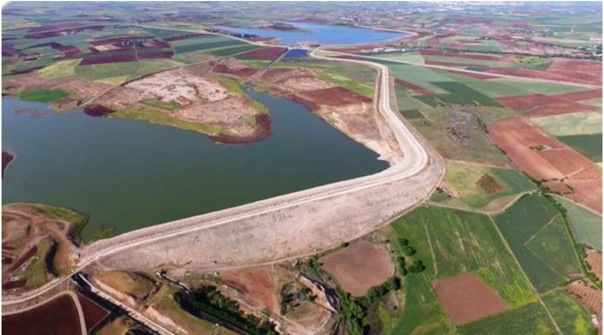
Figure 2. View of Çamgazi Dam ( www.google.com/images ).
