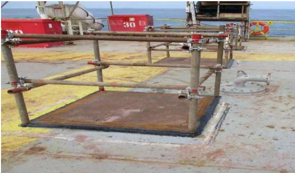
Figure (8): Composite repairs on FPSO main deck plate [67]
