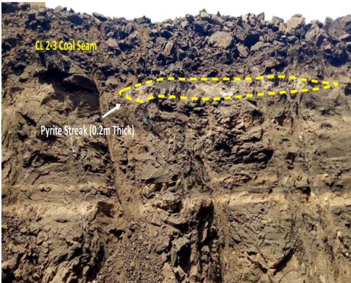
Fig. 03 Localized pyritic streak evident at the top 0.5m portion of CL 2-3 coal seam
