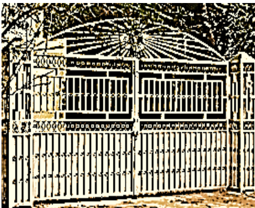
Fig. 4: Gate constructed with simple linear pipes, at Ede road, Osogbo. Photograph: F. M. Abejide, 2020.
