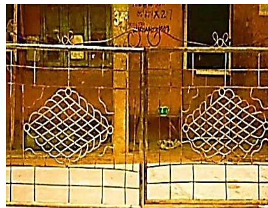
Fig. 5: A see through gate from rods, at No. 34 Catholic Hospital road, Osogbo. Photograph: F. M. Abejide, 2020.
