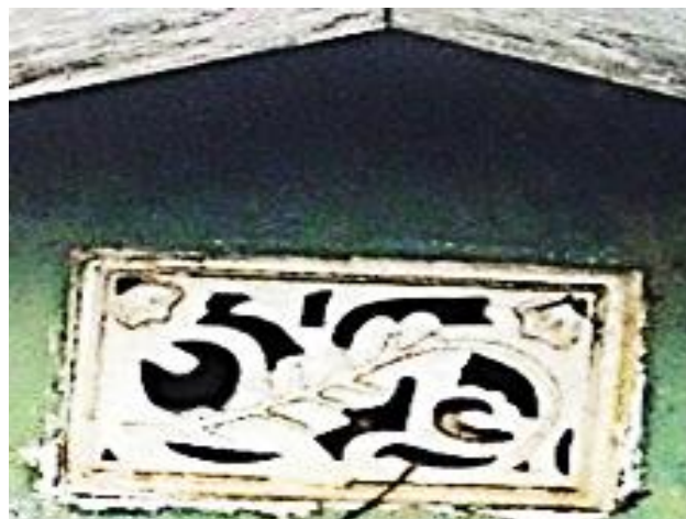
Fig. 2: Prefabricated acanthus leaf pattern in pediment aeration. Photograph: F.M. Abejide, 2020.
