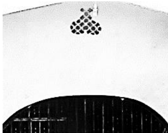
Fig. 4: Pediment with fruit design from arranged stucco blocks, at Onward area, Osogbo. Photograph: F.M. Abejide, 2020)
