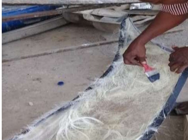
Plate IX: Application of polyester- resin to the fibre
